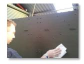
Before starting ensure all surfaces are clean and free from any contaminants. Panel wipe is one good way of achieving this. Ensure you have tested the paint you want to use for the stencil on your vehicles body work for any reactions.
